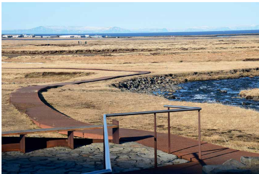
Figure 4. The path designed to make the Svodusfoss waterfall accessible follows a minimalist aesthetic, aiming to have the least possible ecological and visual impact. However, the architectural details are carefully crafted, and the materials have been chosen with care. Even natural patterns are evoked in some way by the path, which mirrors the course of the river and the landscape's morphology. The colours blend into the landscape, remaining visible yet harmonious. The landscape design shows all its consistency and effectiveness here. Along the route to visit Svodusfoss, dry stone walls have been built according to Icelandic building traditions, using stones from the local area. These elements evoke aspects of the local landscape and are integral to the local culture. Seats have been installed on top of them to offer visitors the opportunity to stop and rest, sheltered from the wind, and to enjoy the best and most significant views of the natural monument. Photo by D. Stefano, 2024.
